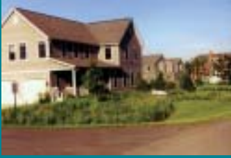
Bioretention with Native Vegetation Prairie Crossing Grayslake, IL
