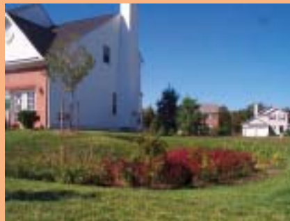
Bioretention Area and Open Space
